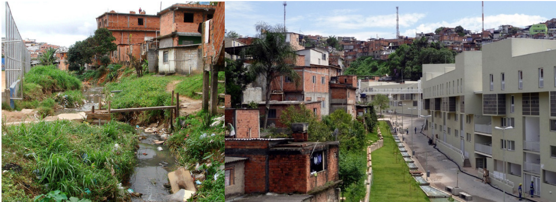
Figure A2: State of the local stream before and after the intervention. Source: Viglicca & Associados, 2012
