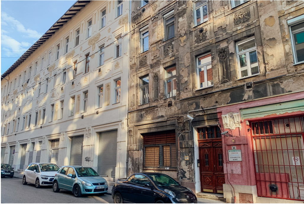
Figure 47: Buildings at Gát Street highlight the heterogeneous character of the area. The distinctions between the two mixed-use buildings within the same complex arise from their conservation status. The structure on the left side of the image has recently undergone renovation, whereas the one on the right awaits refurbishment. Source: by author.
