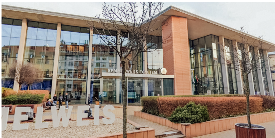
Figure 49: Contemporary aspect of the facade of the Semmelweis College building at Thaly Kálmán Street.
